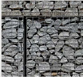
Gabion Wall Application Exterior Cladding
