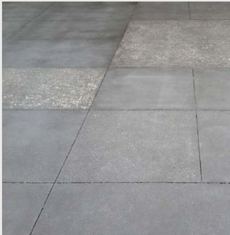
Cast-in-place Pigmented sawcut Concrete
